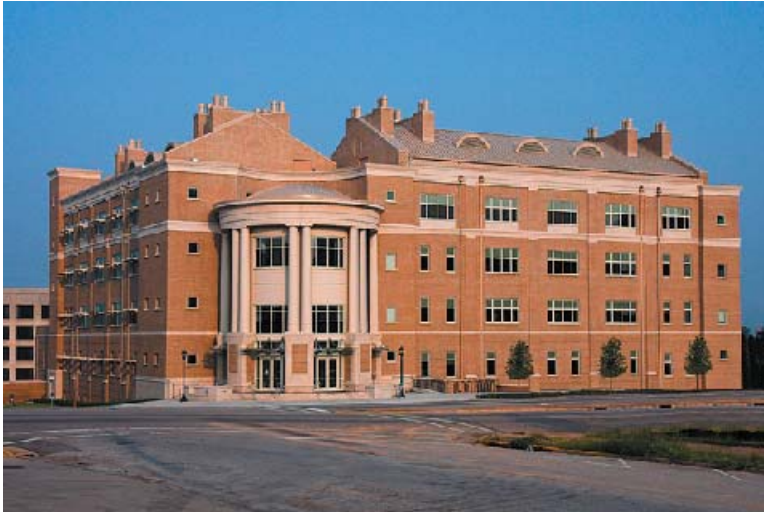
The “new” Public Health Research Building at 921 Assembly Street.
